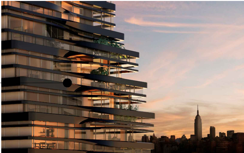
horizontal dark metal cladding
