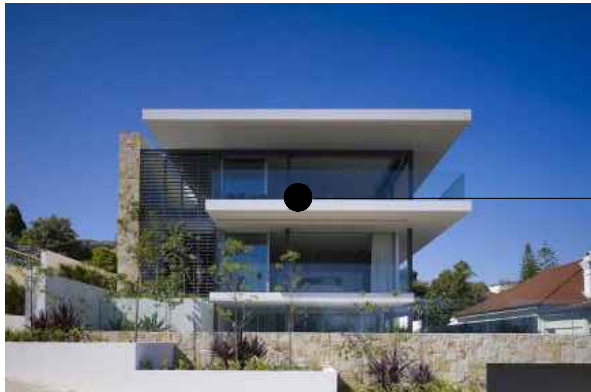
horizontal pattern of white concrete slabs with render
